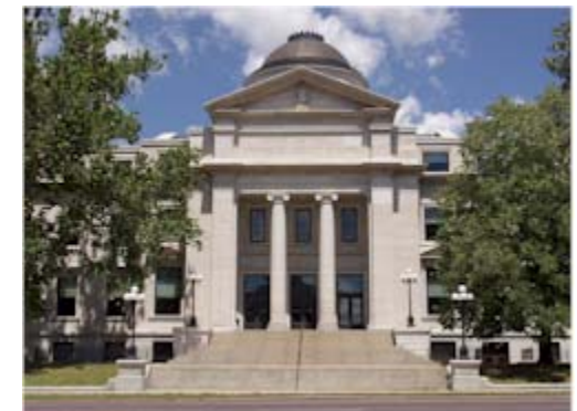
Ola Babcock Miller Building
